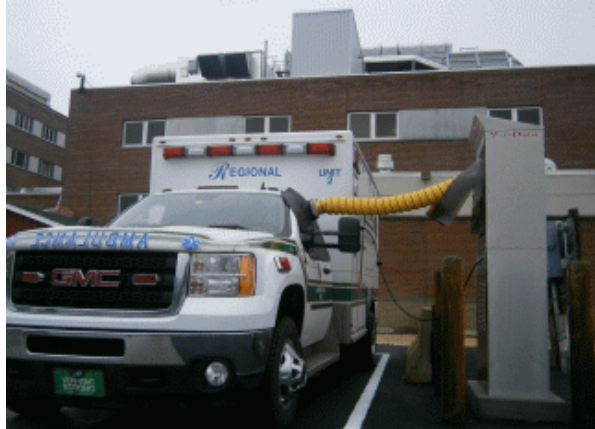
Figure 2: Ambulance connected to MediDock EPS Kiosk (HVAC and power). Courtesy of Vermont Department of Environmental Conservation.
