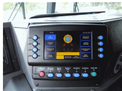
Figure 4: Diesel APU IRT system control panel. Courtesy of United States Air Force, HQ Air Force Civil Engineer Center (AFCEC)/CXF, Tyndall Air Force Base.
